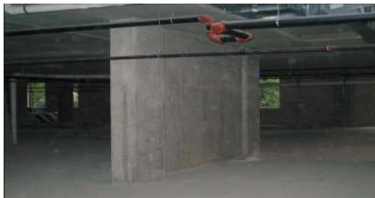
Fig2. Construction of shear wall
