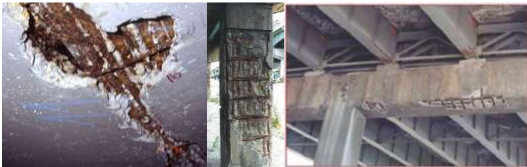
Fig.1. Corrosion of Steel Reinforcement in Structures
