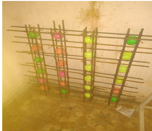
Fig -6: Location & placing of hollow balls
