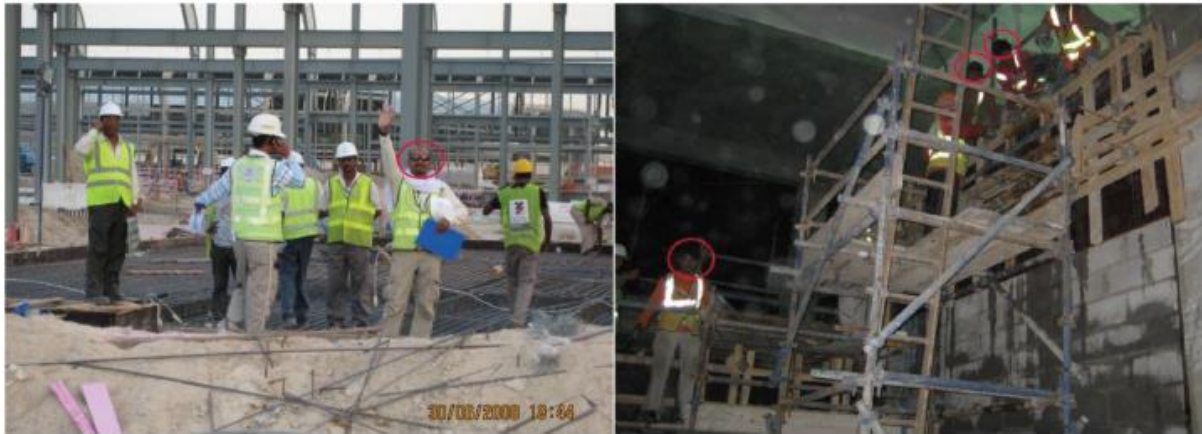
FIGURE 1: A typical construction site where some workers did not use hard hat and some used it improperly.
