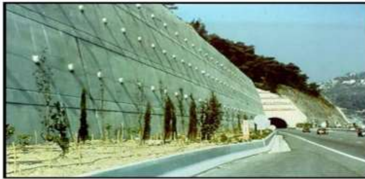
Figure 1.1.3 application to soil nailed walls
