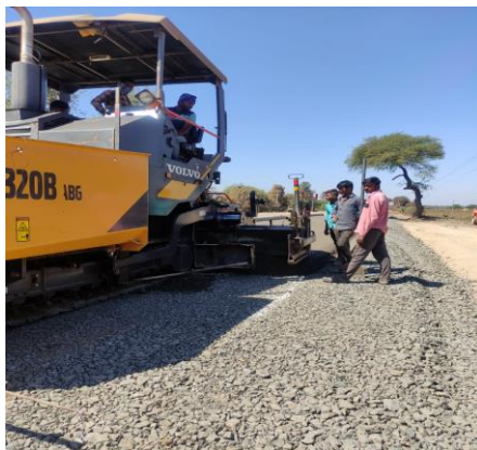
Fig. 4 Levelling and Compaction of Road
