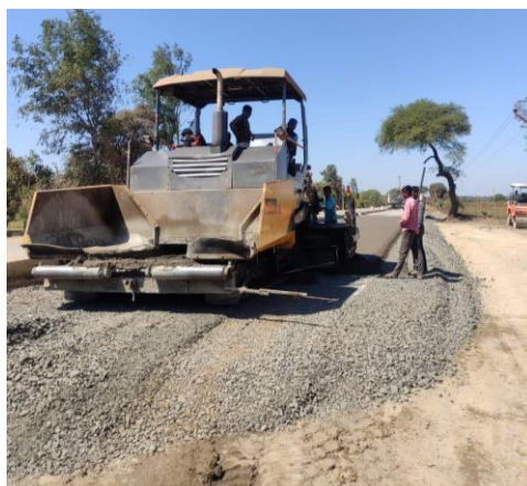
Fig. 3: Shows Maintenance work By Paver Machine
