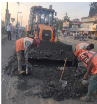
Fig. 2: Selected site for Maintenance work
