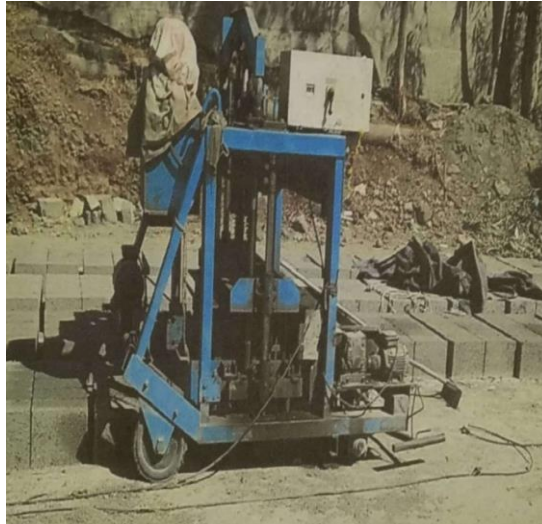
Fig-3 Manufacturing of Compressed Stabilized Earth Blocks
