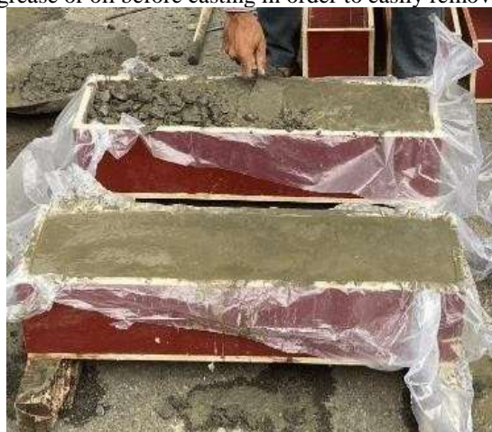
Fig 4 Casting of Beam Panels
