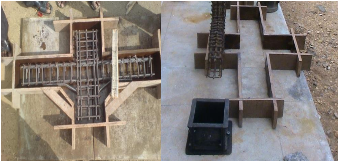
Fig 2&3: Details of formwork
