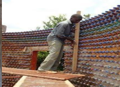
Fig .2: Fixing of bottles with wooden
