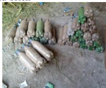
Fig.1: Fill Plastic bottle with sand
