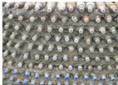
Fig -3: Plastic bottle wall
