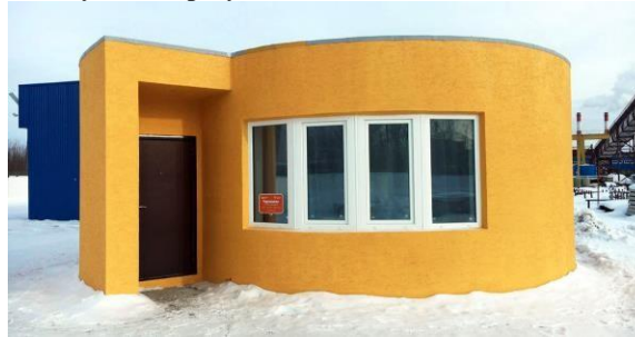
Fig 2 Apis cor 3D printed building
